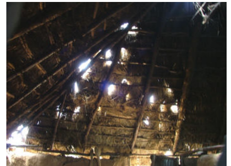
Holes in the roof - where the rain gets in.
