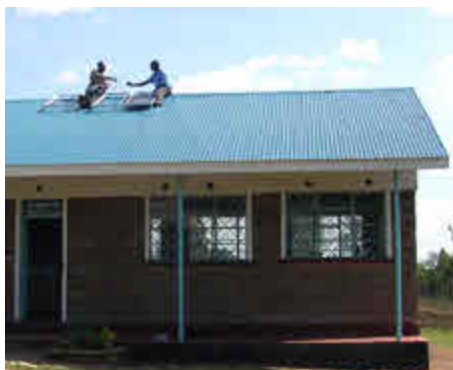
Electricians installing solar power
